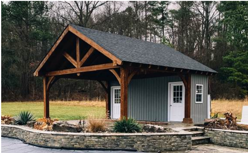
14x20 A-frame pool house with vinyl board & batten enclosed area, timberwood pavilion deck, shingle roof, 3' fiberglass 9 lite single doors, 24x36" vinyl insulated windows & walnut stain
