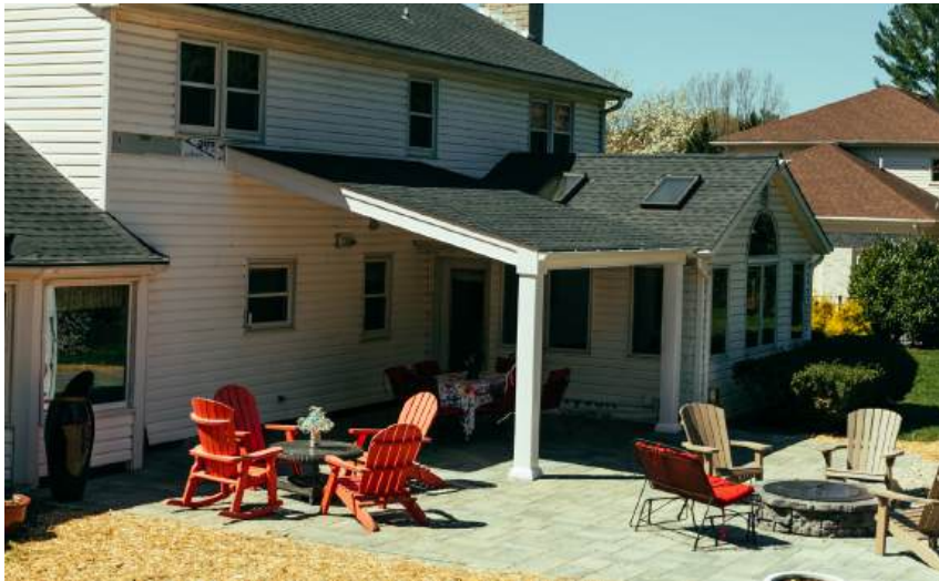
16x18 attached vinyl lean-to with shingle roof & modern post trim
