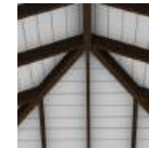
Ceiling unfinished T&G & exposed rafters pine T&G or nickel gap LP smooth panel cedar paneling vinyl beadboard
