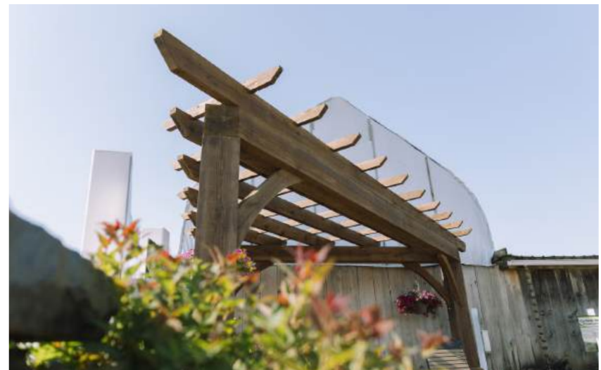
Custom triangular timberwood pergola made with rough-hewn hemlock
