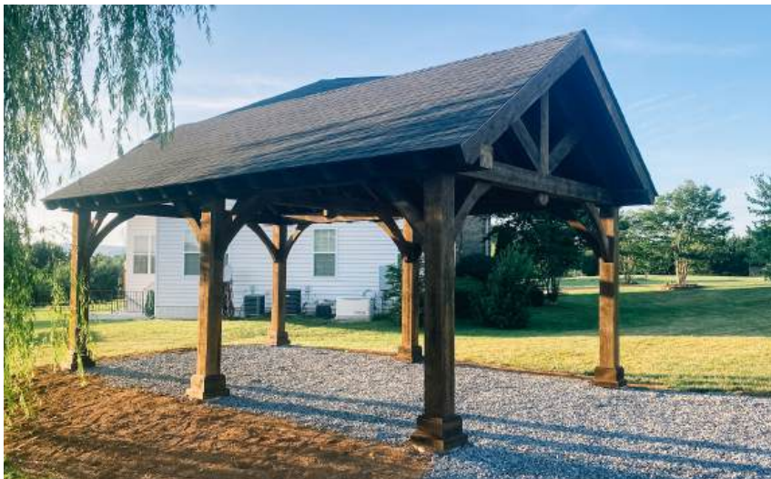
14x20 timberwood A-frame, open gables with braces, shingle roof & walnut stain
