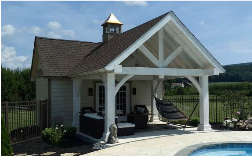
Custom timberwood A-frame with shingle roof, exposed rafter ceiling, 10x10 posts & beams, white stain & attached studio enclosure
