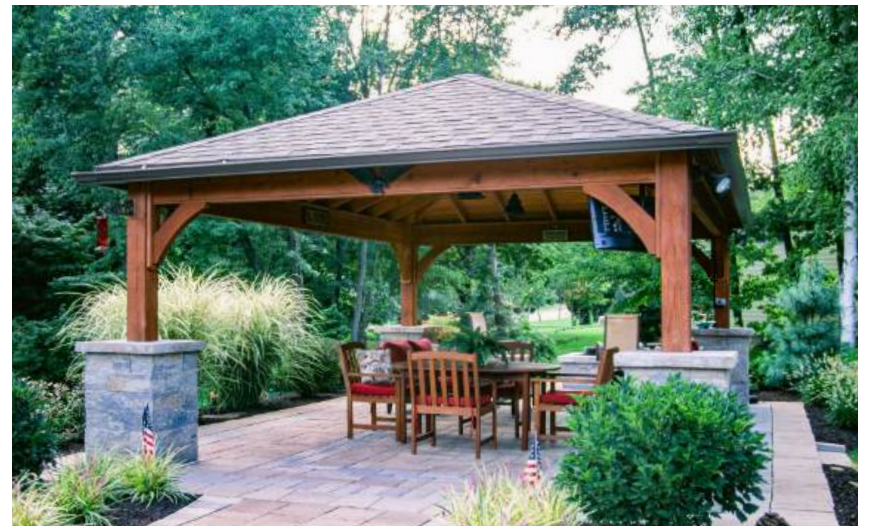
16x16 wood hip with shingle roof, exposed rafter ceiling, traditional post trim & mahogany stain
