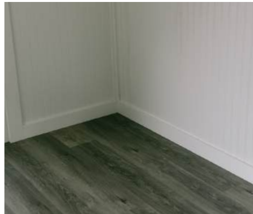
Vinyl plank interior flooring
