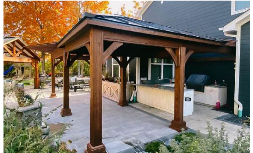
Custom attached wood hip with standing seam metal roof, traditional post trim, custom classic pergola attachment & rustic cedar stain
